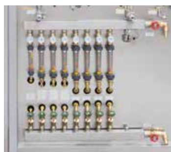
Cooling water distribution
