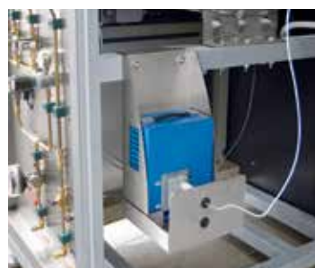
Acid pump for nitric acid
