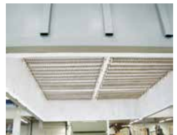
Heating elements in furnace hood
