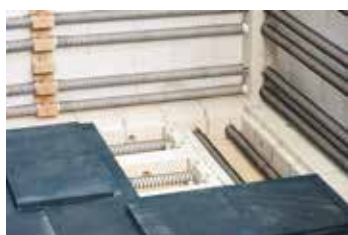
Bottom heating covered by SiC tiles to create level stacking support
