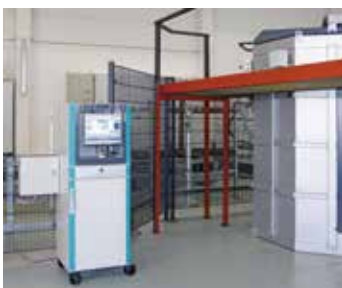
PC interface for central furnace operation
