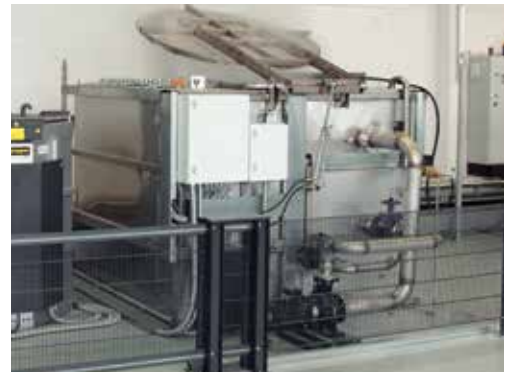
Quench tank with water integrated in a tempering plant for aluminium
