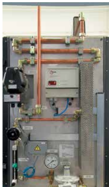
Sophisticated gas supply system
