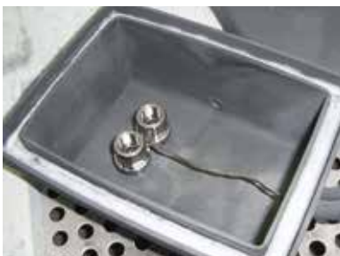
Brazing in a gas-supply box
