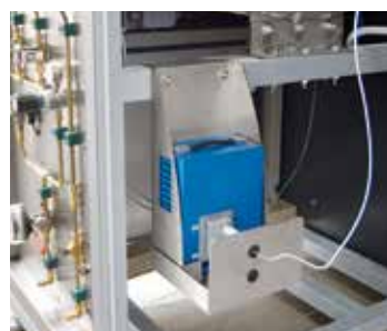
Acid pump for nitric acid
