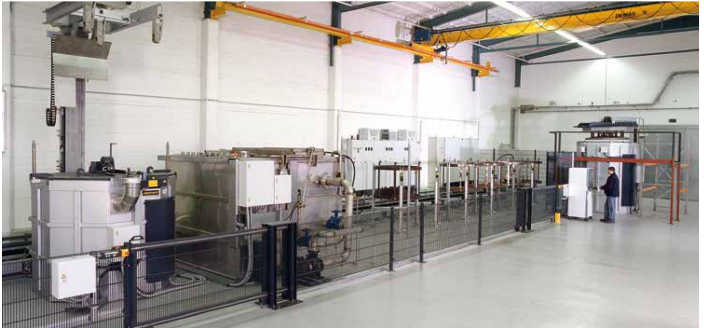
Fully automatic tempering plant for aluminum with 2 pit-type furnaces, water bath, and 6 parking places
