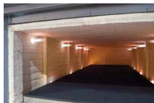
Furnace chamber with eight high-speed burners
