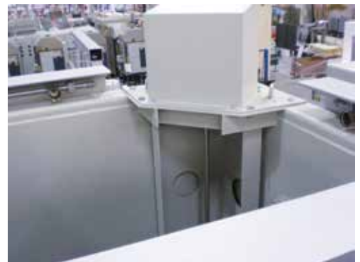
Protective gas supply as fire protection
